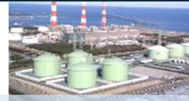
Maintain stockpile systems
